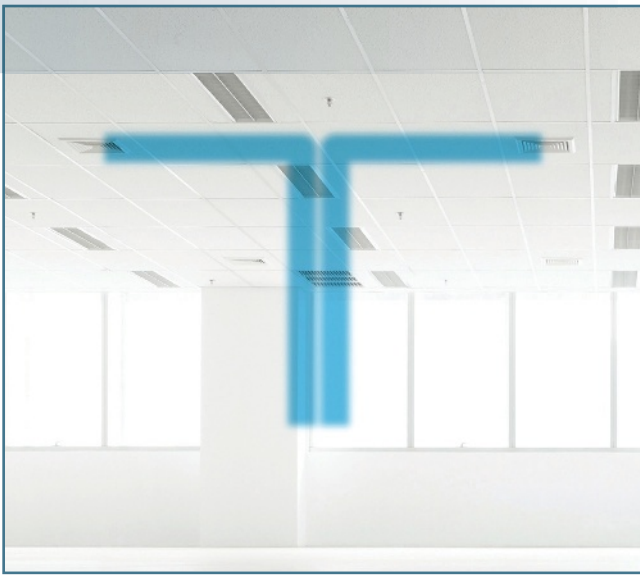
PHOTOS 1A AND 1B. Based on the ratio of isothermal throw at 50 fpm (0.25 m/s) to the midpoint between diffusers, ADPI aids design for comfort. An ADPI of 80 percent or greater indicates a space is well-mixed and that drafts and stratification are unlikely. If ADPI is less than 80 percent, occupant discomfort and complaints can be expected. Above, on the left, is an illustration of optimal ADPI; on the right is an illustration of poor ADPI.
