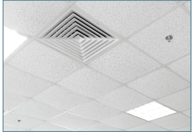
PHOTO 4. Square diffuser installed in a closed ceiling. innoom/Shutterstock
